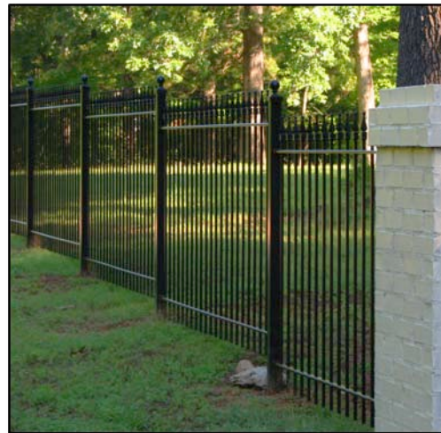
Figure 13 - Stair Stepped Fence Panels
