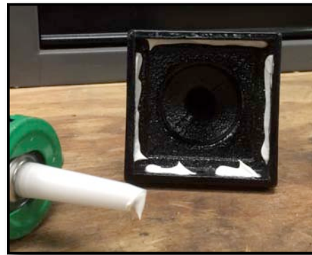
Figure. 15 - Apply Under the Cap
