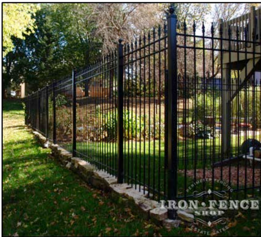
Figure 12 - Backfilled with Stones
